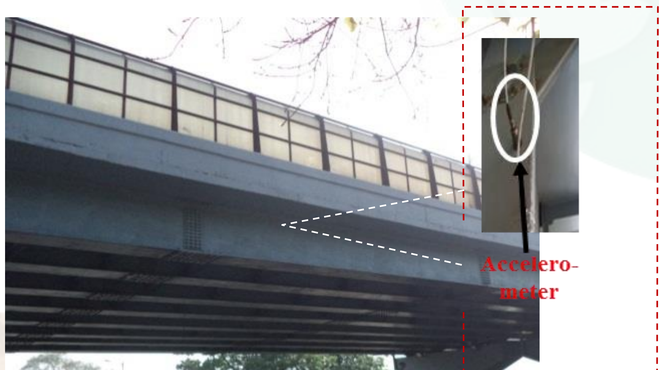
Fig. 1 Deployment of accelerometer on girder
