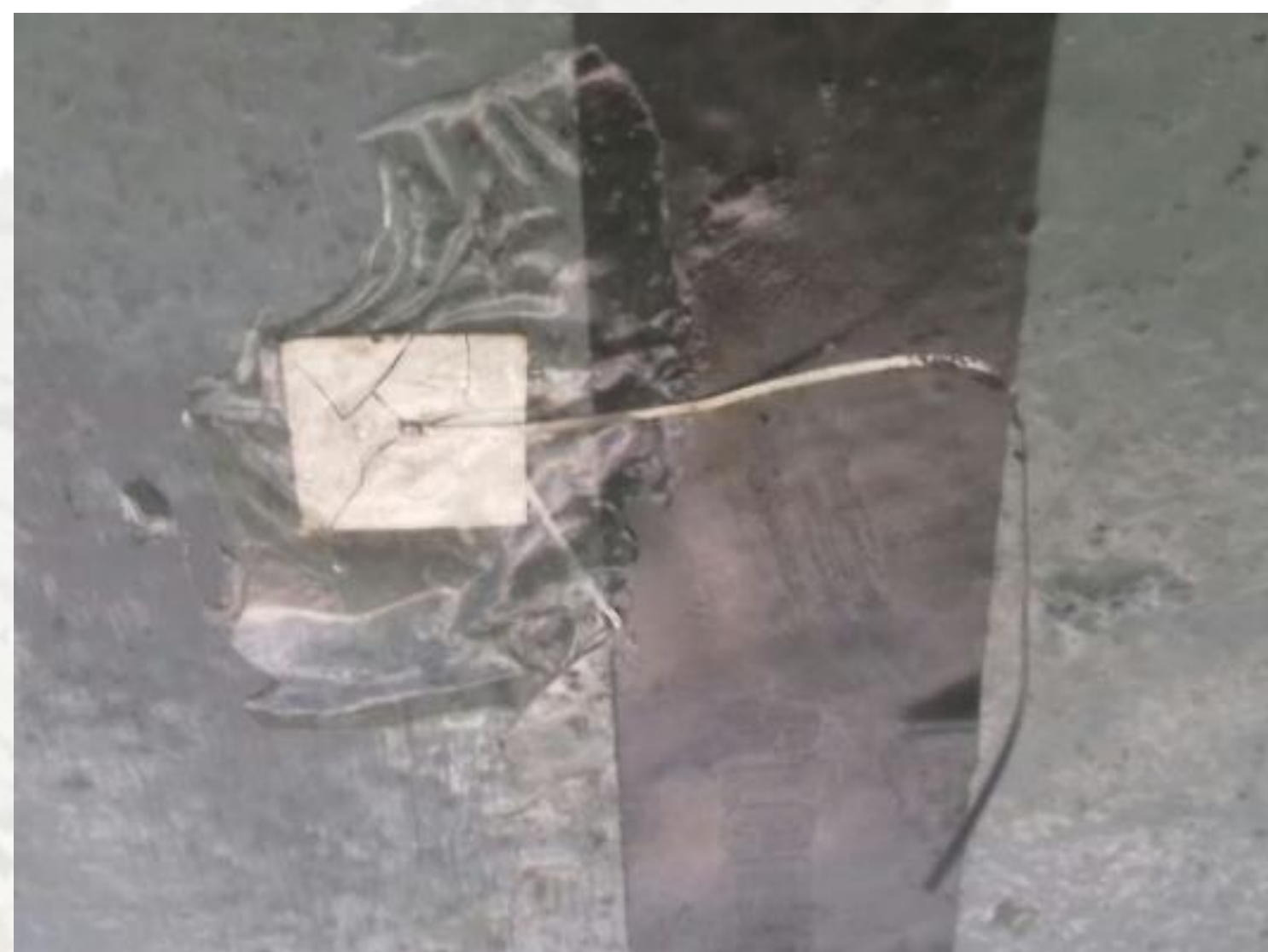
Fig. 6 Close up of PZT bonded on girder.
